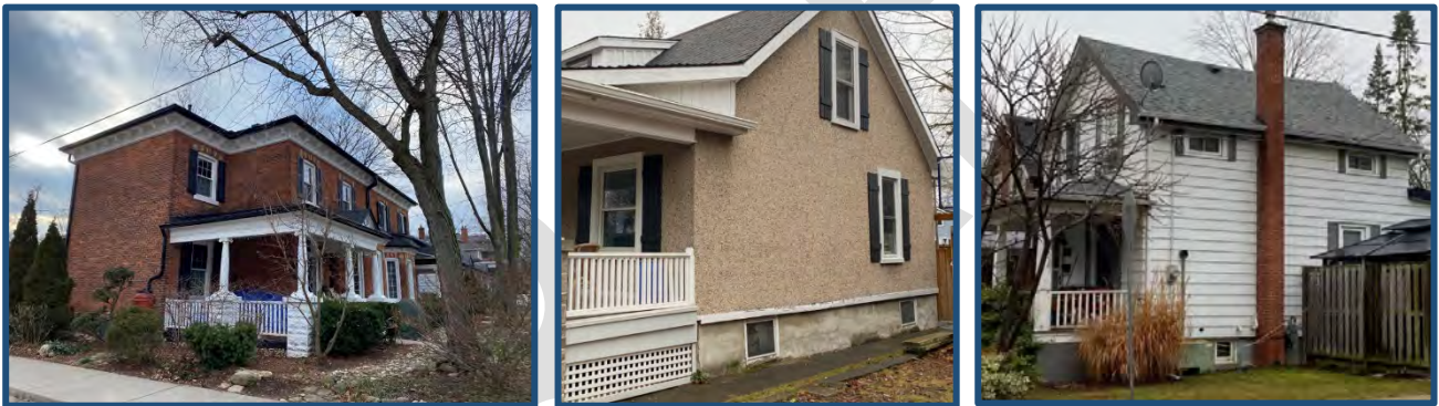
Photos 30-32 - (left) Example of a red brick dwelling; (middle) Example of a pebbledash stucco clad building; (right) Example of a building clad with synthetic siding (Source: MHBC, 2023)
