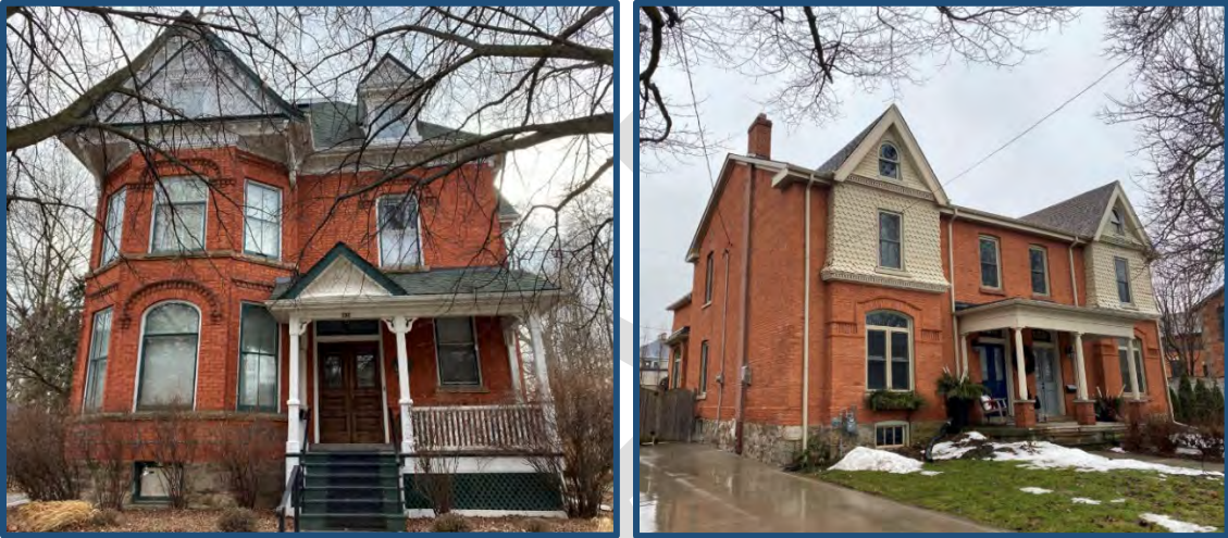
Photos 25 & 26 - (left) Example of a Queen Anne dwelling located at 132 Melville Street; (right) Example of Queen Anne semi-detached dwelling located at 100-102 Park Street West (Source: MHBC, 2023)
