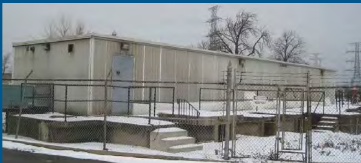
Water Treatment Plant Substation (Constructed late 50's)
