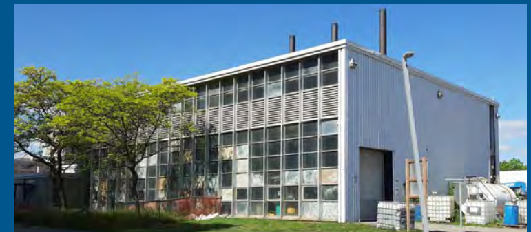
Standby Power Facility (Constructed early 70's)
