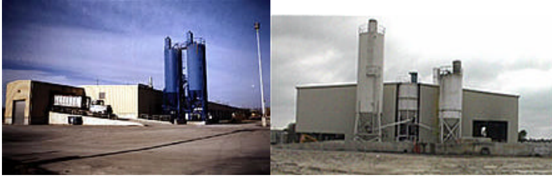
Figure 12: Photo Examples of Alkaline Stabilization Facilities
