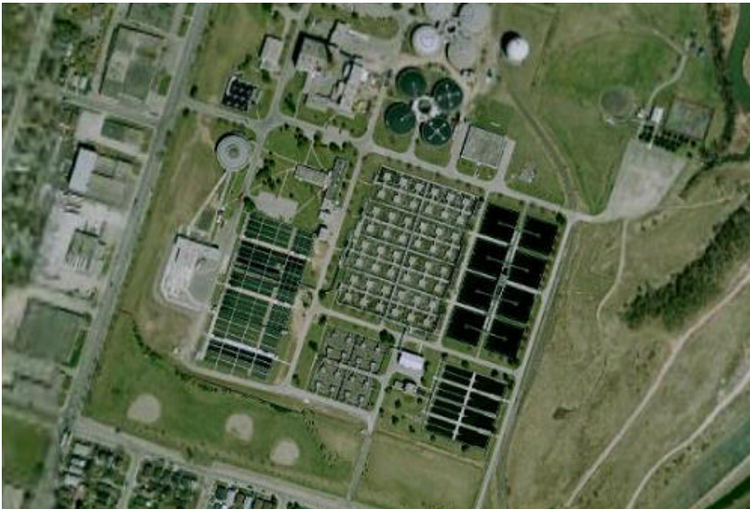
Figure 1 Aerial View of the Woodward Avenue WWTP
