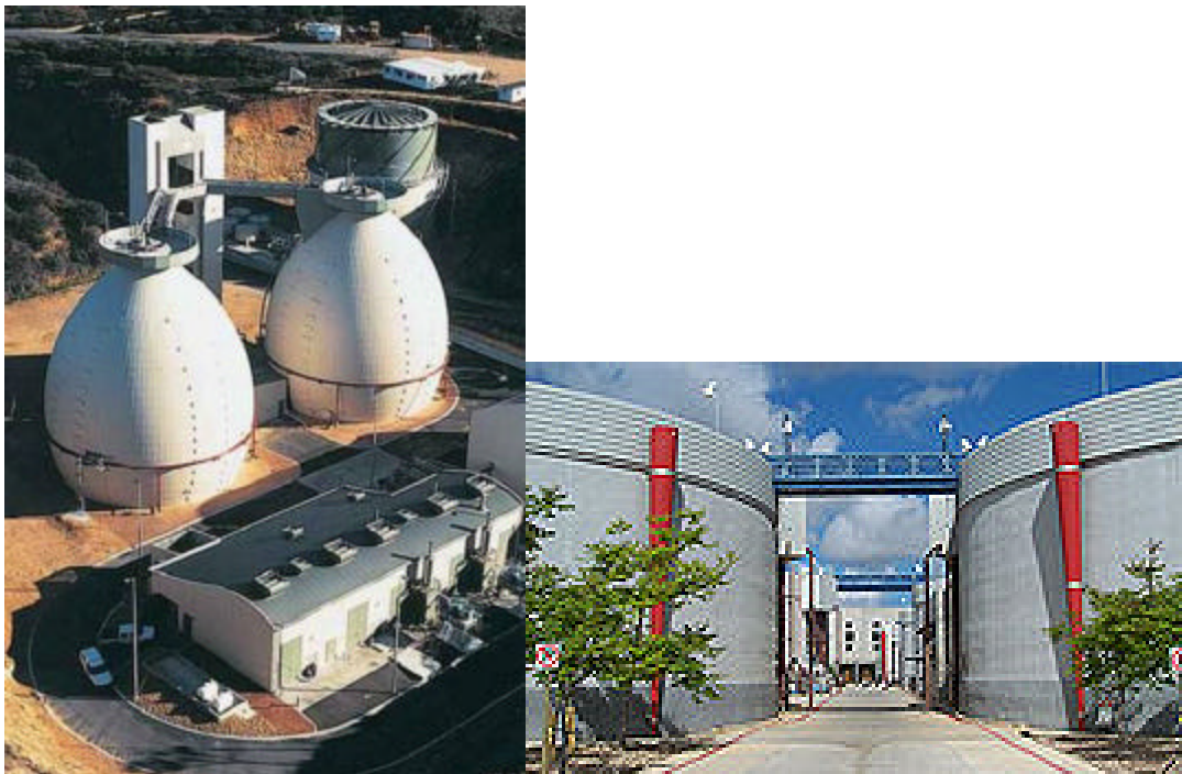
Figure 11: Photo Examples Of Anaerobic Digesters
