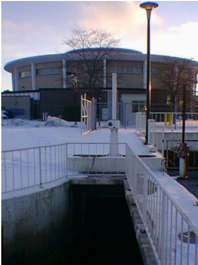
Figure 4: Woodward Avenue WWTP
