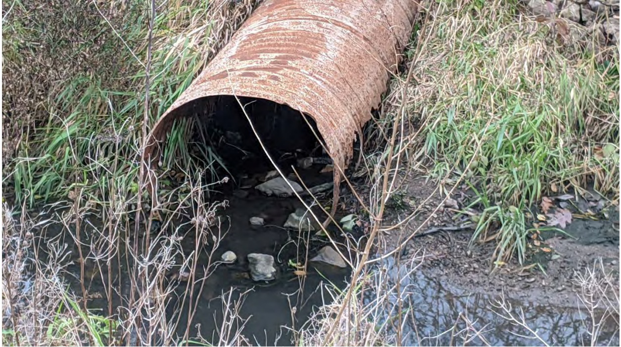
The 1600 mm Culvert that outlets to Red Hill Creek also appears to be in very poor condition.
