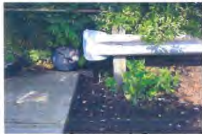
Small Channel Maintained by Local Residents
