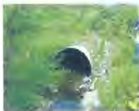
Outlet of 1600 mm \phi Pipe at South End of Berm
