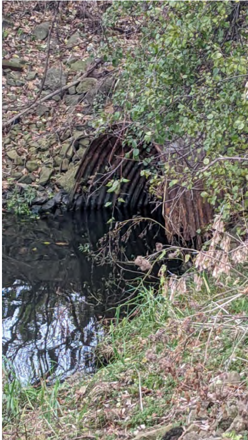
The 1600 mm Culvert that outlets to Red Hill Creek also appears to be in very poor condition.
