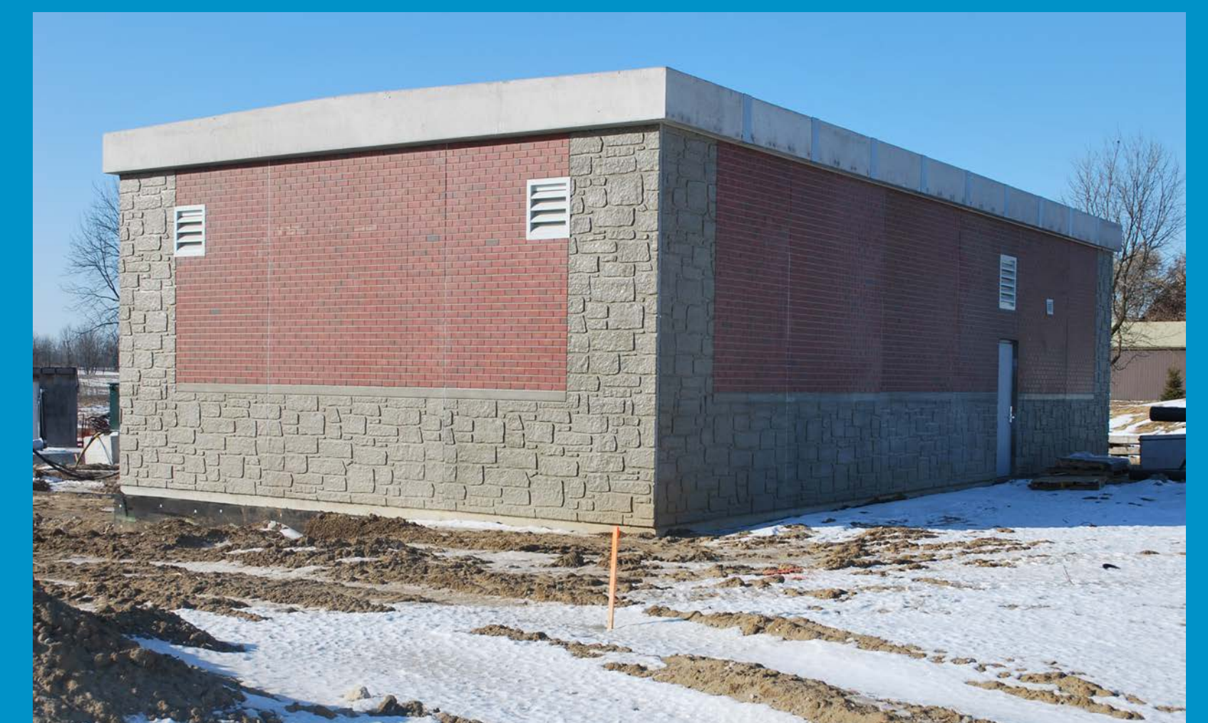
New treatment plant building
