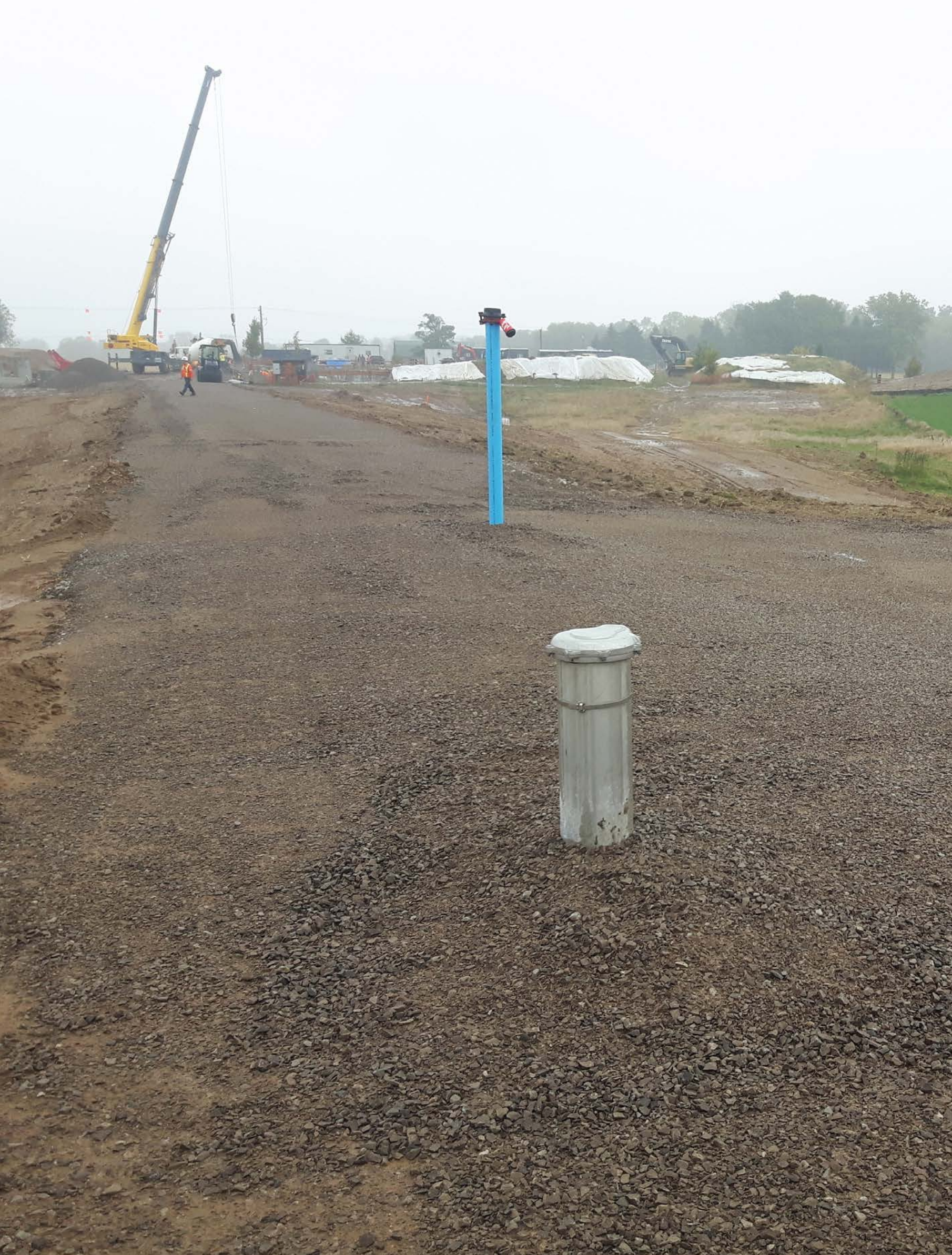
New access road and new municipal well
