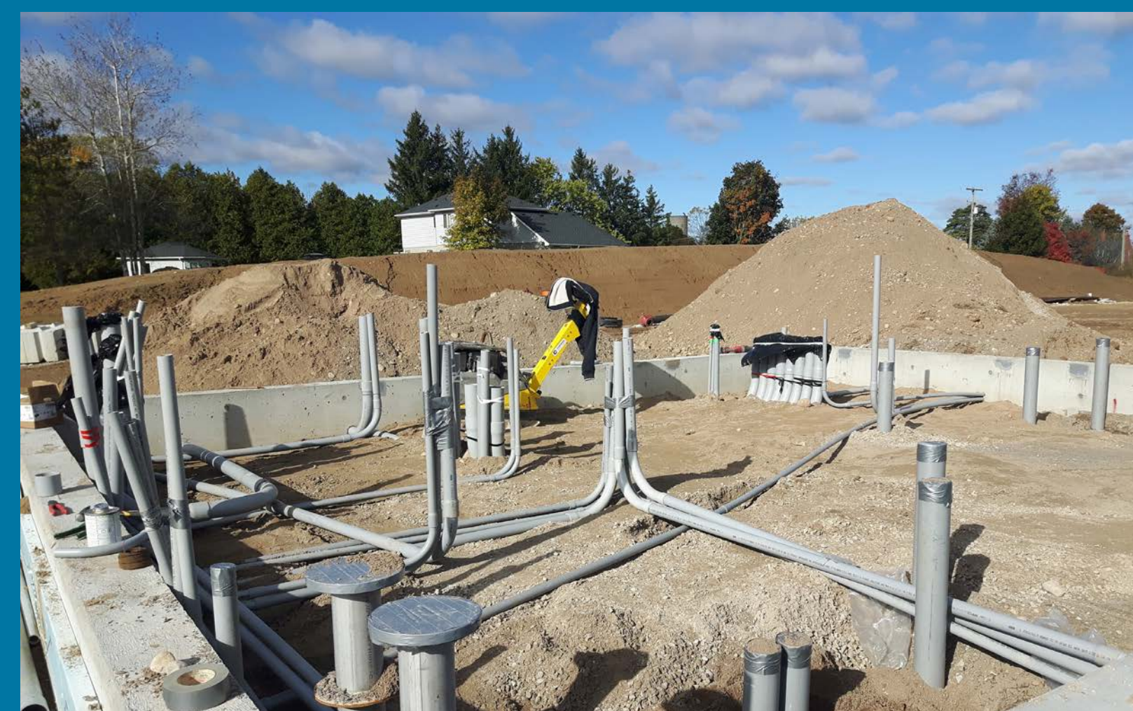
New plumbing and electrical conduit before floor slab is poured
