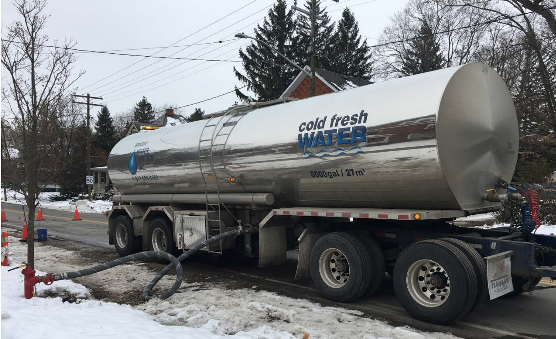
Tanker truck connected to a flushing hydrant with a hose
