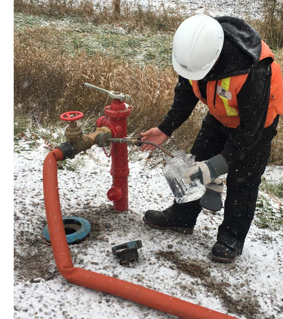
A flushwater sample being collected from a flushing hydrant
