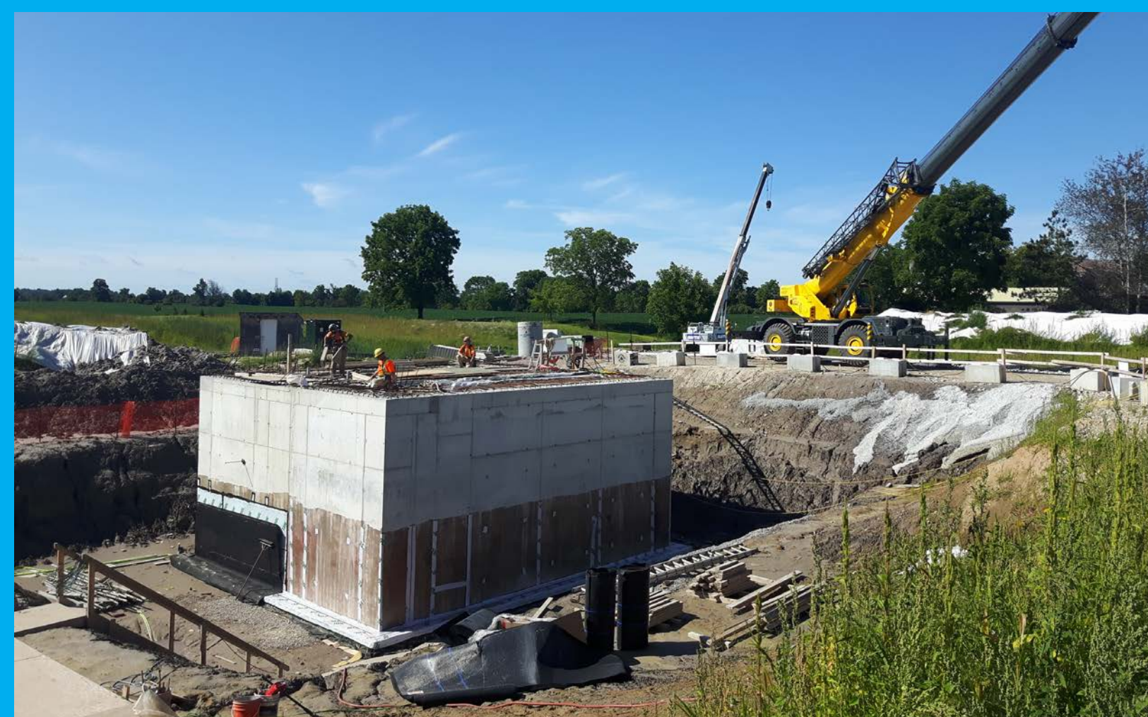
New reservoir under construction
