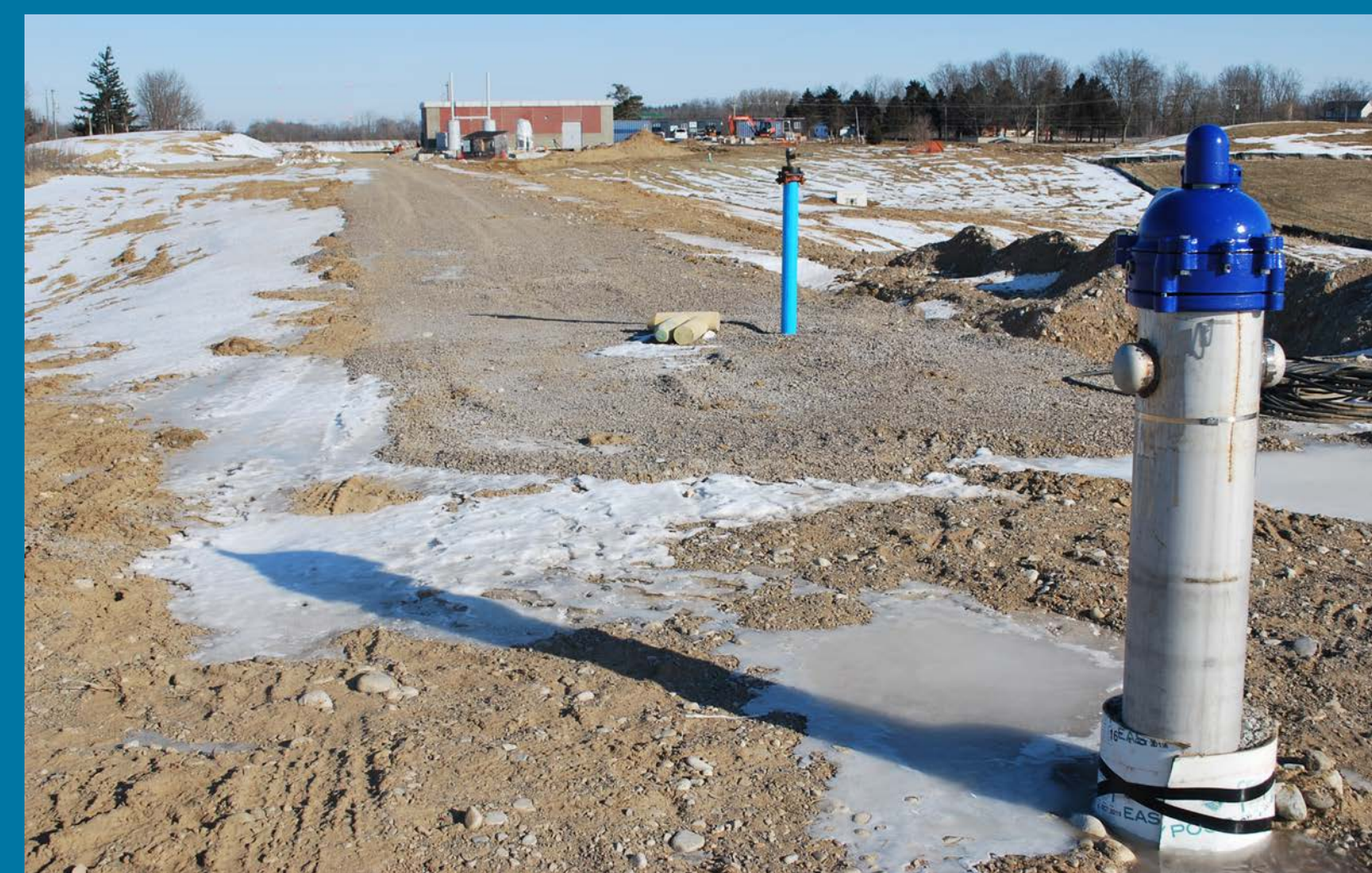
New access road and municipal well FDL03
