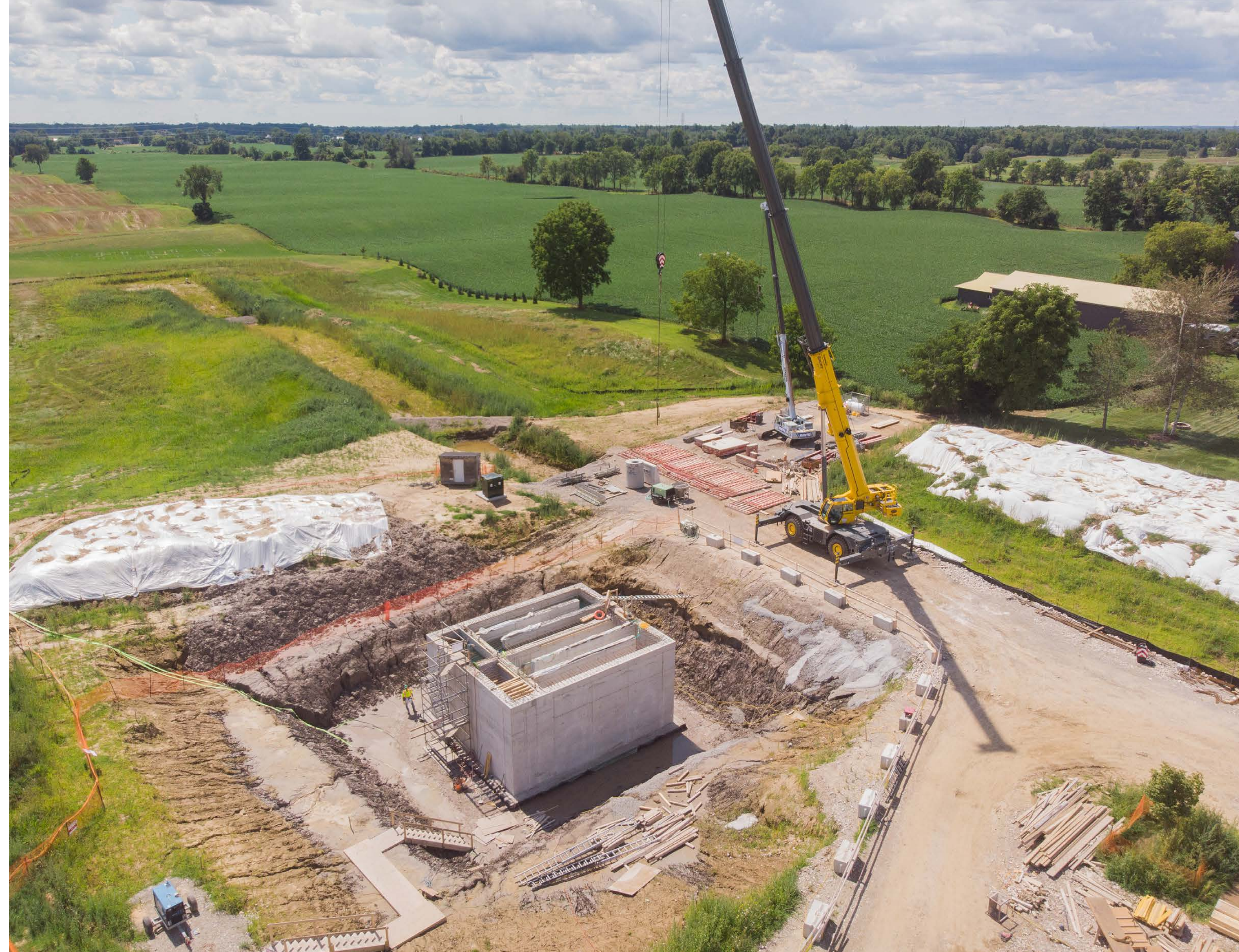
Aerial of new reservoir
