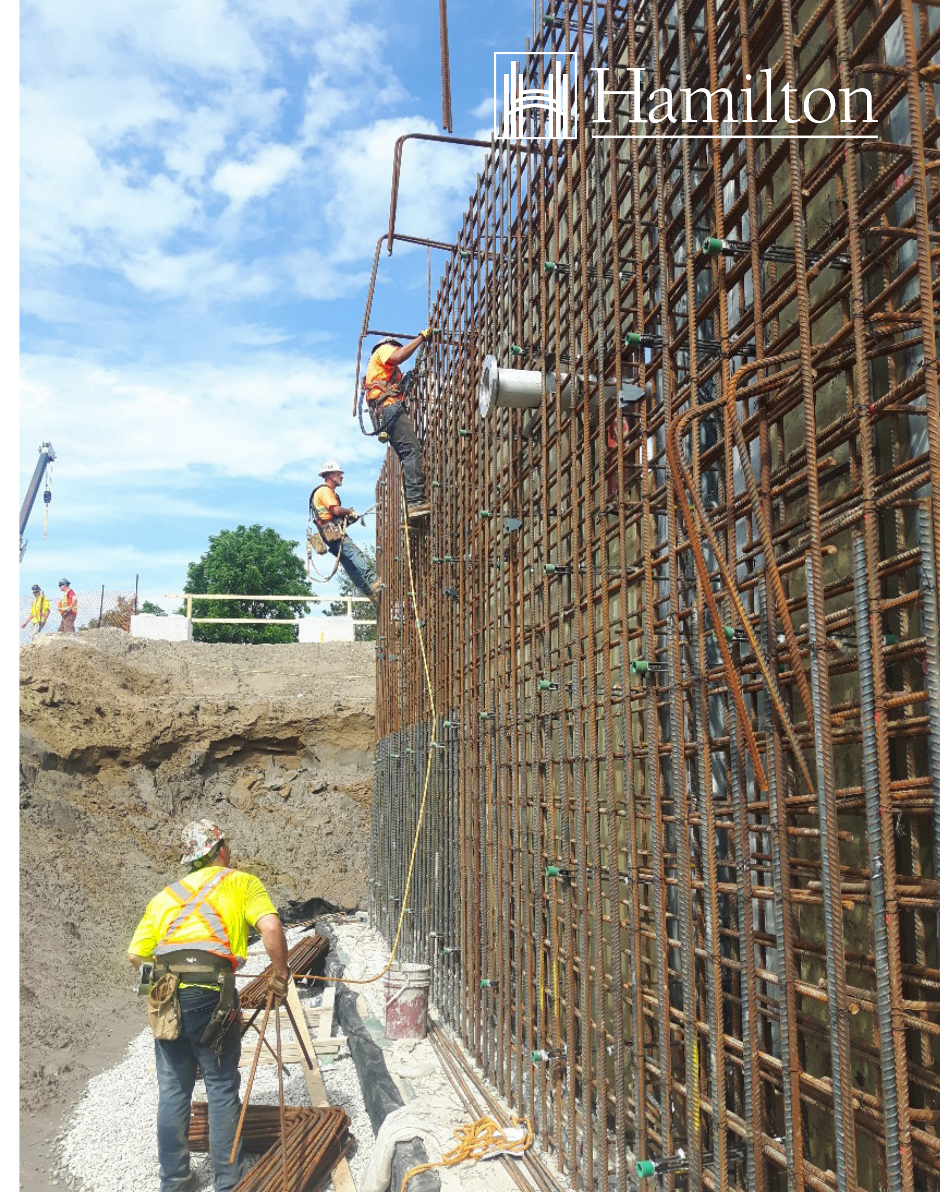
Rebar installation for the new reservoir
